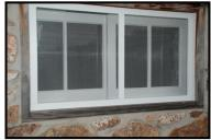
Most recently (Fall 2020) five new windows (two-unit) with screens were installed, and one window (two-unit) was refurbished and reinstalled with a screen in the lower level of the granary. In addition to the new windows, a
